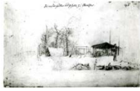
Early Ebenezer Shelter structure
