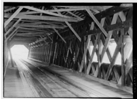
Watson Mill Bridge, Historic American Engineering Record Library of Congress, Prints & Photographs Division, HAER GA-140
