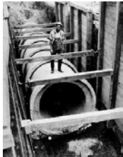
Orme Street relief sewer, WPA Collection
