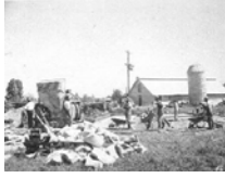
Nancy Creek sewer project, WPA Collection
