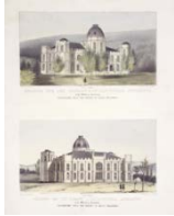
Library at West Point
