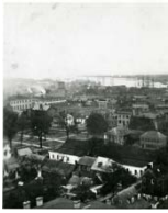
St. James Square, Telfair Square 1
