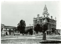
St. James Square, Telfair Square 2
