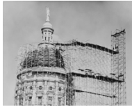
Dome Restoration Courtesy of Georgia Archives, Small Print Collection, spc19-036e
