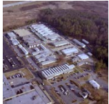
Areal view of Chamblee GA CDC campus 1988 Courtesy of the Centers for Disease Control and Prevention
